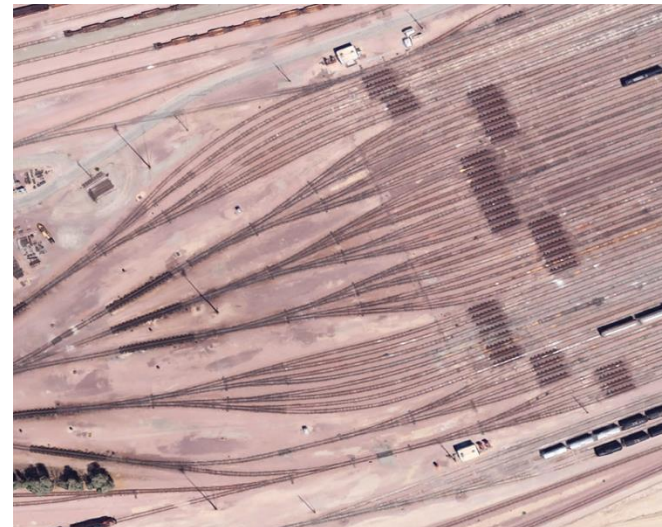
Railroad Switch Station
