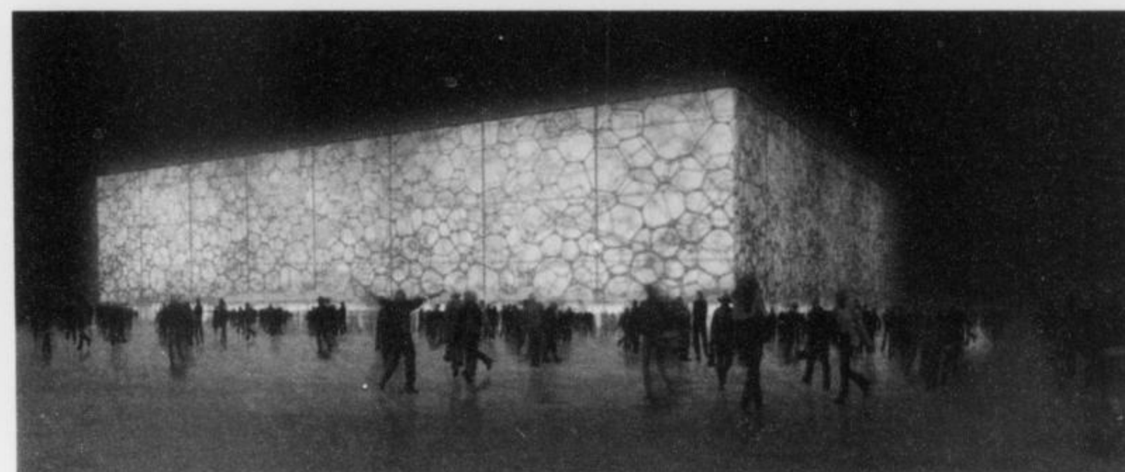
Figure 5. The architect's vision of the "WATER CUBE" (in the foreground) in front of the main stadium. The award-winning design of the National Swimming Centre for the Olympic Games in 2008 in Beijing is based on the Weaire-Phelan structure. It was developed by consulting engineers Arup and partners, PTW Architects, the China State Construction and Engineering Corporation, and the Shenzhen Design Institute, who provided the image.
